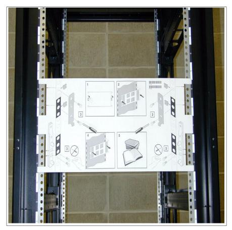
Figure 3-2 Template positioned on rack flange
