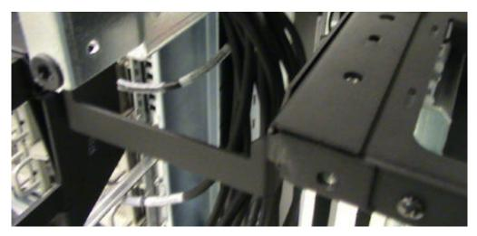
Figure 4-7 Rack Bonding Spacer – Top of Rack
