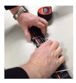
Figure 1-54 Pull Apart the Cable Management Arm
