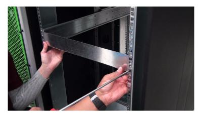
Figure 1-15 Adjustment Using the Alignment Tool
